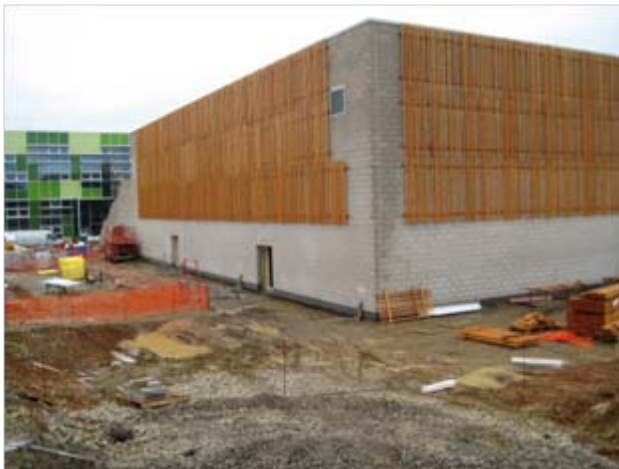
Sports hall (cladding works)
