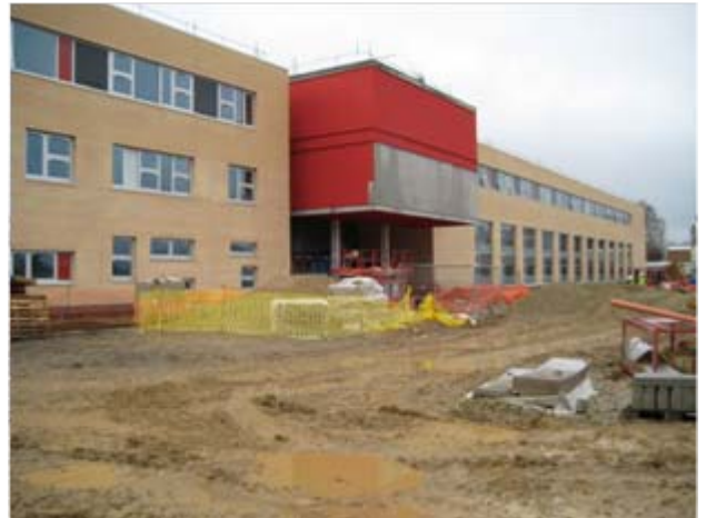
North elevation (main entrance to the school)
