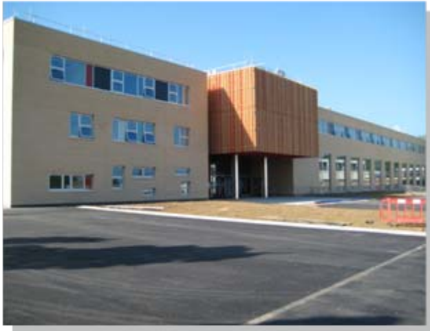
North elevation (main entrance to the school)
