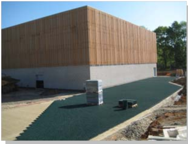
Sports hall (cladding and grasscrete works)
