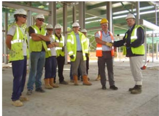
Photo of H.Young Structures being presented with a £50 voucher by Carillion's Project Manager, Andy Beavis, for the monthly 'Don't Walk By' safety award.
